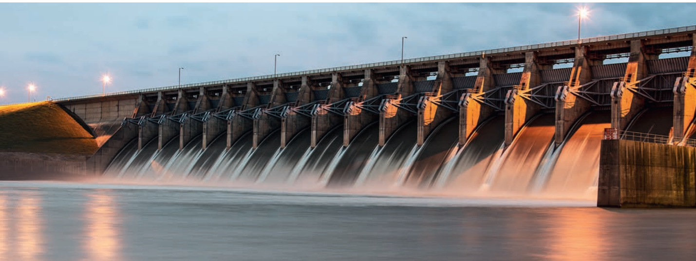
Dam with spherical plain bearings in the tide gates
